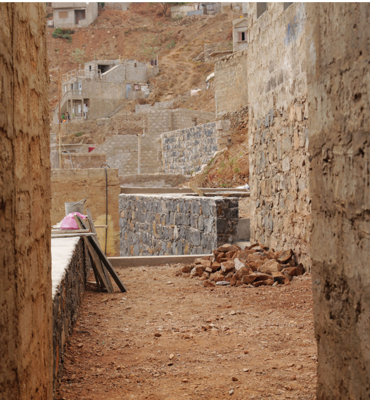
Obra do projeto Pontual 3, 2021 / IOB Construction, Phase 03, 2021.
